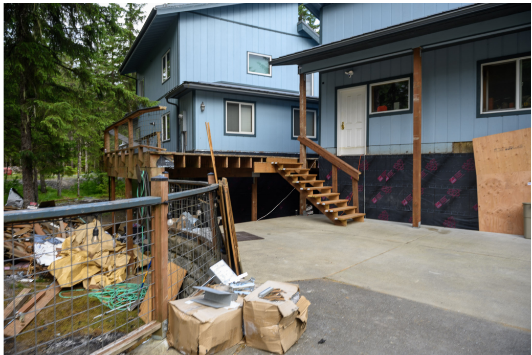
Stairs lead up to the home of the Winters on View Drive on July 11, 2026. The house has been raised by nine feet over the years. (Jasz Garrett / Juneau Independent)
