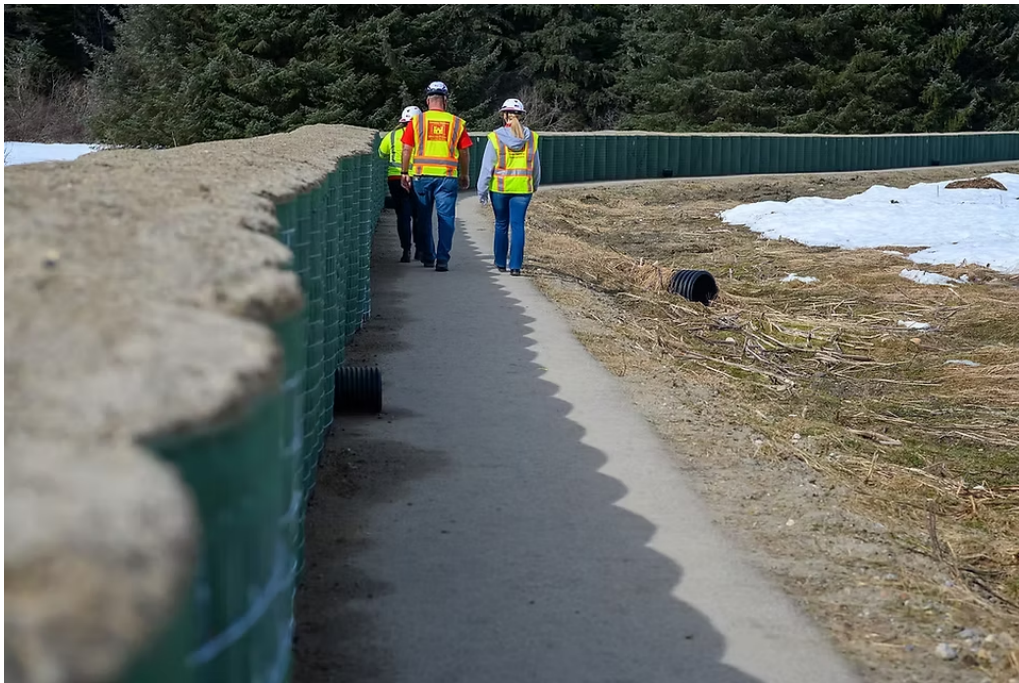
U.S. Army Corps of Engineers members from its Emergency Operations team walk near HESCO barriers installed by Brotherhood Bridge on April 15, 2026. (Jasz Garrett / Juneau Independent)
