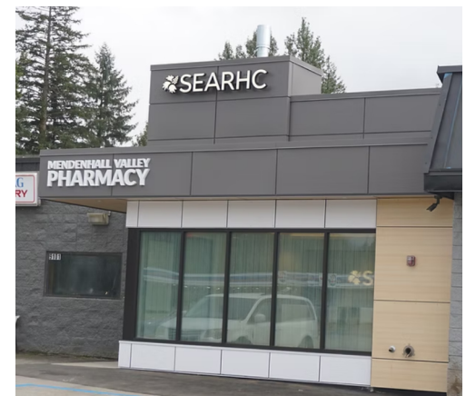
The new SEARHC pharmacy in the Mendenhall Mall on Tuesday, Aug. 18, 2026. (Ellie Ruel / Juneau Independent)
