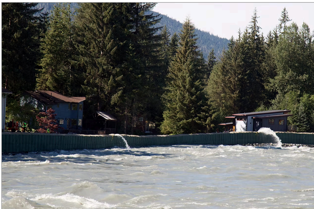
Pumps push water over HESCO barriers near River Road as the Mendenhall River reaches its crest of 14.7 feet at about 2:15 p.m. Thursday, Aug. 13, 2026. (Mark Sabbatini / Juneau Independent)
